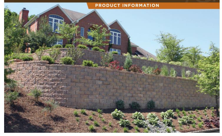
Tall walls and tight spaces don't mean sacrificing visual appeal for structural integrity. The Vertica Stone Cut® retaining wall system lends even the most massive projects the warmth and character of rough-hewn textures and earthen tones. And as always, with a 4-degree batter, the Vertica Stone Cut product rises to the challenge of creating walls of virtually any height while maximizing valuable land.
